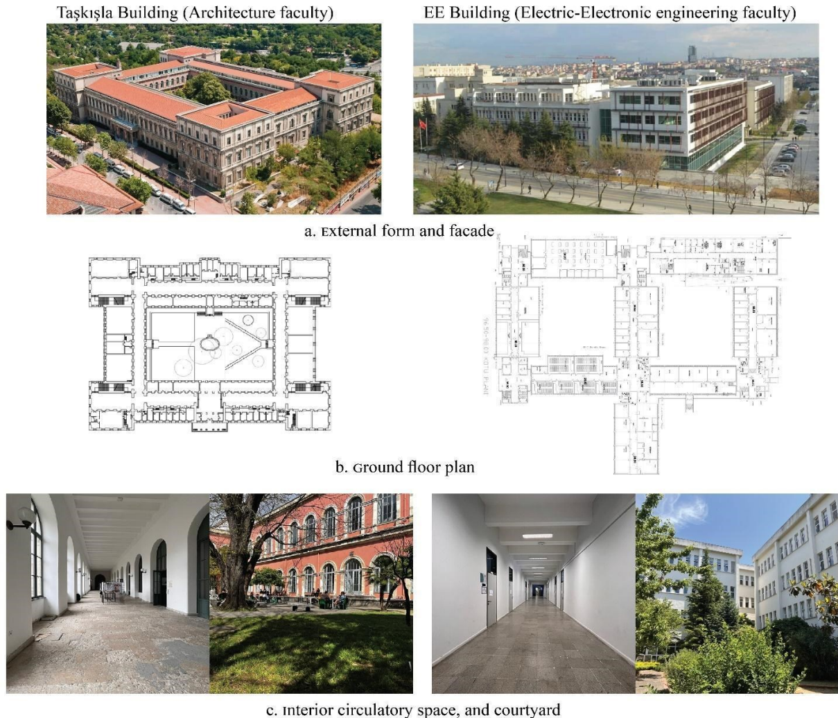
Figure 4. The two faculty buildings that were used for the comparative method.
