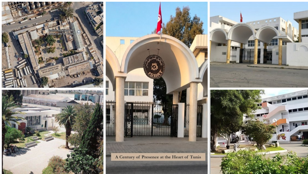
Figure 4. ISBAT Architectural Morphology and Urban Context: Spatial Configuration, Accessibility, and Integration within the Urban Network of Tunis (Developed by the Author).
