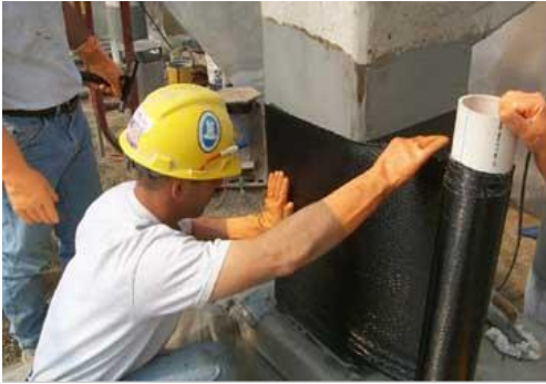
Fig. 7: shows the repair of concrete column with ACM.
