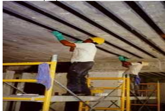
Fig. 6: shows repair of concrete beams with ACM.
