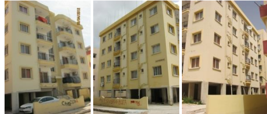
Figure 4. From left to right. West, North, South façade of the Muçize apartment (research's field study, taken by author, 2016).
