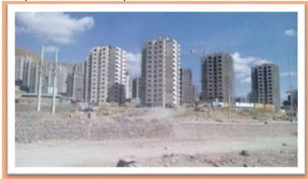
Figure 5: Pardis Mehr housing in suburbs area (URL 4).
