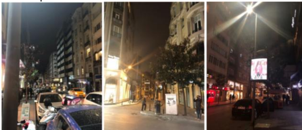
Figure 9. Inadequate Lighting (photo by authors)
