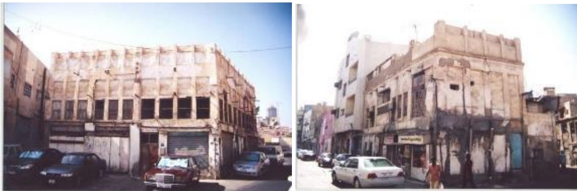
Figure 19. Haphazard car parking with low level of maintenance.
