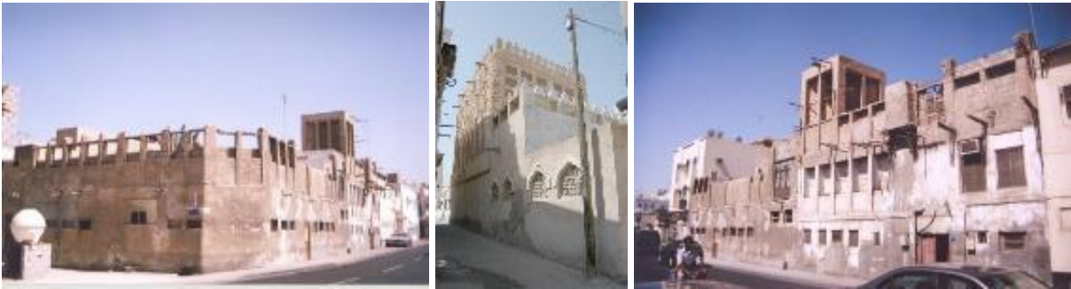
Figure 20: Deteriorating traditional building condition (air conditions are haphazard disrupted).
