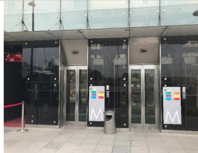
There are many elevators that link the closed garage's floors clearly.
