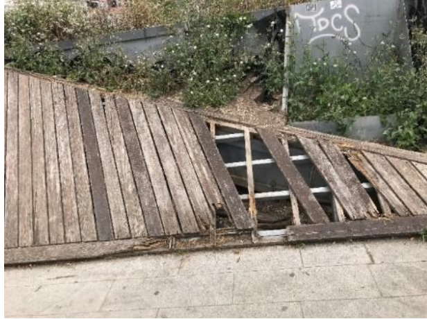
The quality of the used wood materials in the park is very poor and needs maintenance.
