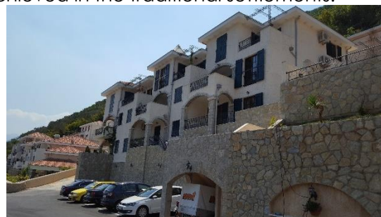
Figure 9. Excessive height of the new building and the retaining walls (Source: Kosara Kujundzic)
