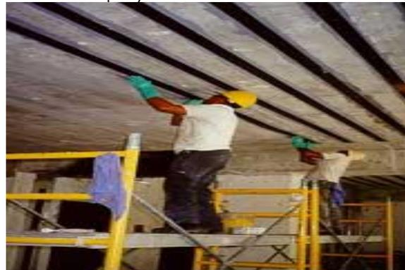
**Fig. 6:** shows repair of concrete beams with ACM.
