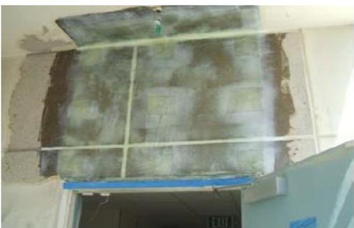
Fig.7: depict the use of advance composite in the healing of concrete spall on wall ([Chiewanichakorn & Toranzo, 2011](#)).
