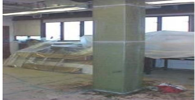
Fig.8: Depict the use of advance composite in the healing of concrete spall on wall ([Chiewanichakorn & Toranzo, 2011](#)).
